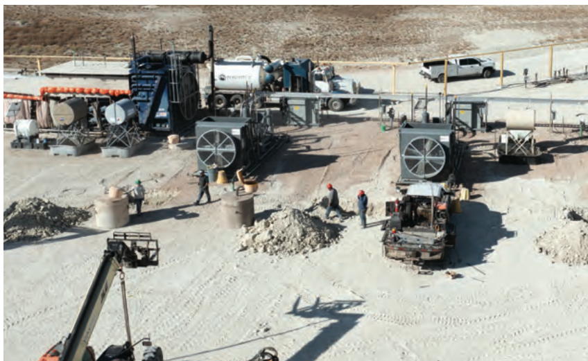
Figure 7: A Fundare production site in Redtail where the transition from gas-fired to new electric-drive compressors is in progress.
