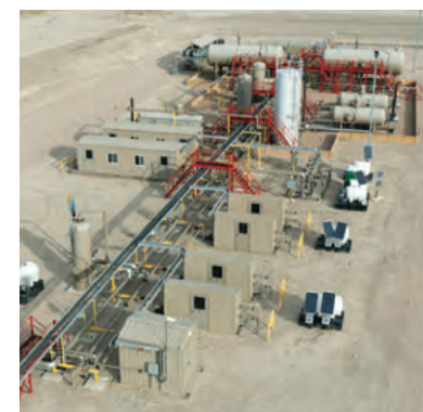
Figure 6: One of Fundare's new construction production sites in the Redtail field with the tankless design.
