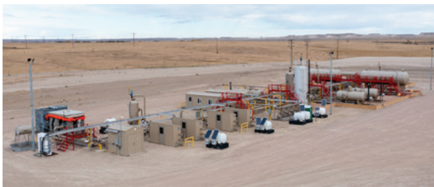
Figure 6: One of Fundare's new construction production sites in the Redtail field with the tankless design.
